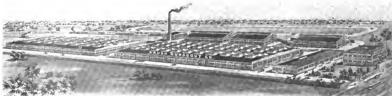
New Home of Brush Runabout Company, Detroit, Mich., with 200,000 Feet Floor Space, Covering 38 Acres
